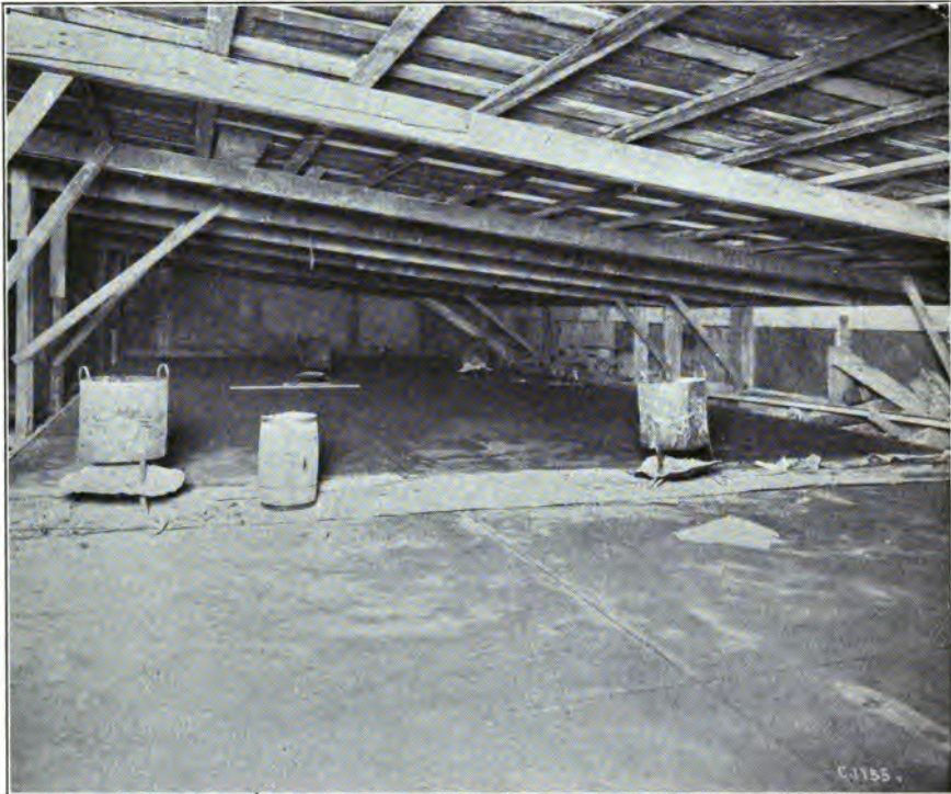
FIG. 11.—SALAMANDERS IN USE ON FINISHED FLOOR.
